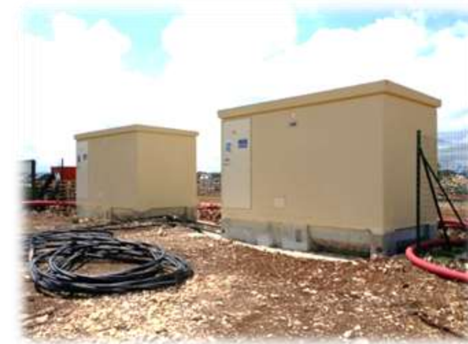
Pose de postes HTA
